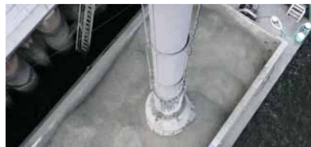
Loading of FGD plaster (400 t/h, l=30m)
