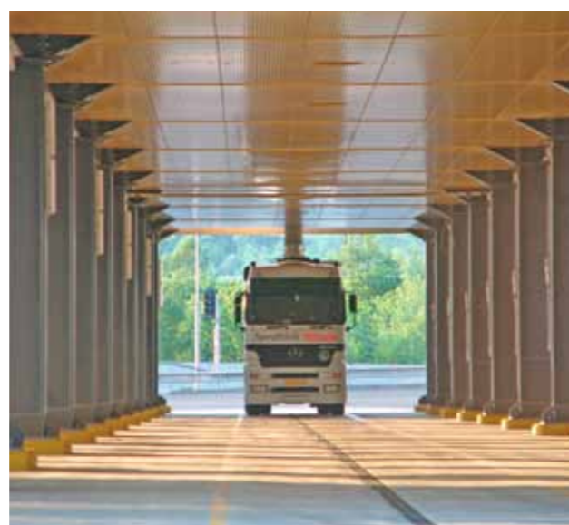
Loading station below MWV-level
